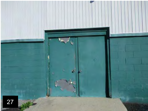
Service Doors with Peeling Paint
