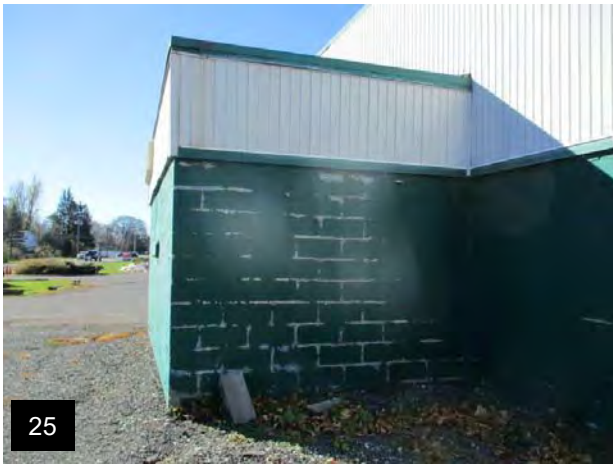
Peeling Paint Along Rear Elevation
