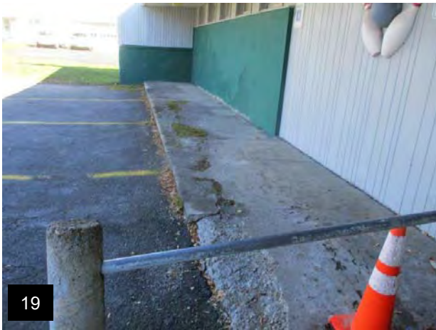
19 Front Concrete with Spalling
